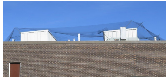
Figure 5. Netting to exclude pigeons from a roof area.
