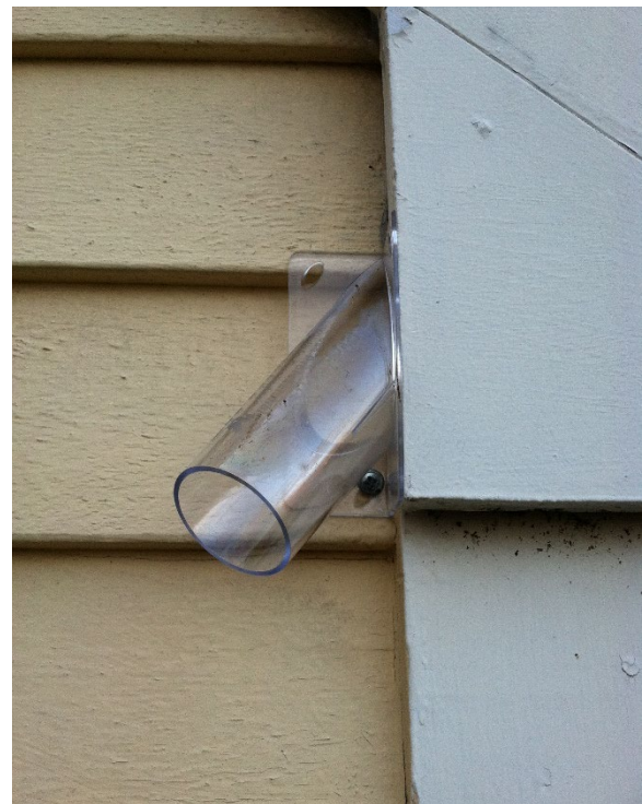
Figure 7. One-way plastic valve which allows bats to leave a structure but not to reenter.
