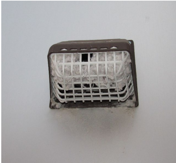
Figure 4. Note the potentially dangerous lint build up on this screened dryer vent.
