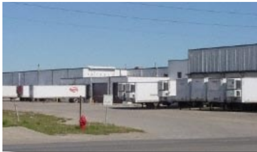
Warehouses can receive multiple shipments simultaneously through their loading docks..
